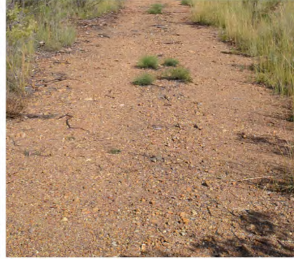
LOCAL GRAVEL AND GRASS NATURAL PATH, BINGARA
