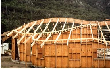
•Durability - As an architect, considerations in specifying a material for sustainability must extend beyond application, to service or how long will it last; the material must then be detailed so that it will last as long as possible. At Brambuk, the architects specified Australian White Cypress. It is a Durability Class 1 material that is highly termite and fungus resistant.
